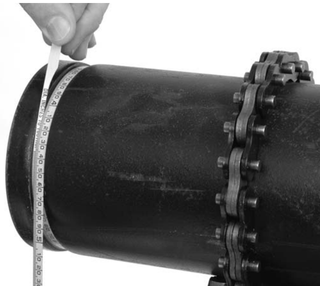
Figure 11 – Checking Groove Diameter With A Diameter Tape
